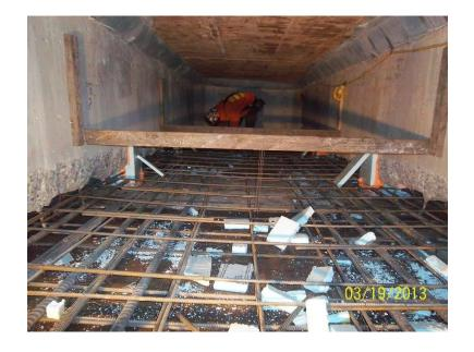
Formwork for new concrete had to be supported by the same vertical elements that supported the temporary support system
