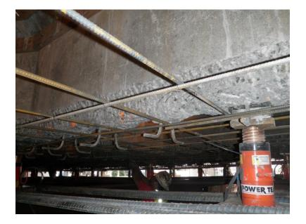
New reinforcing steel in place. Starting to place formwork for square fillets
